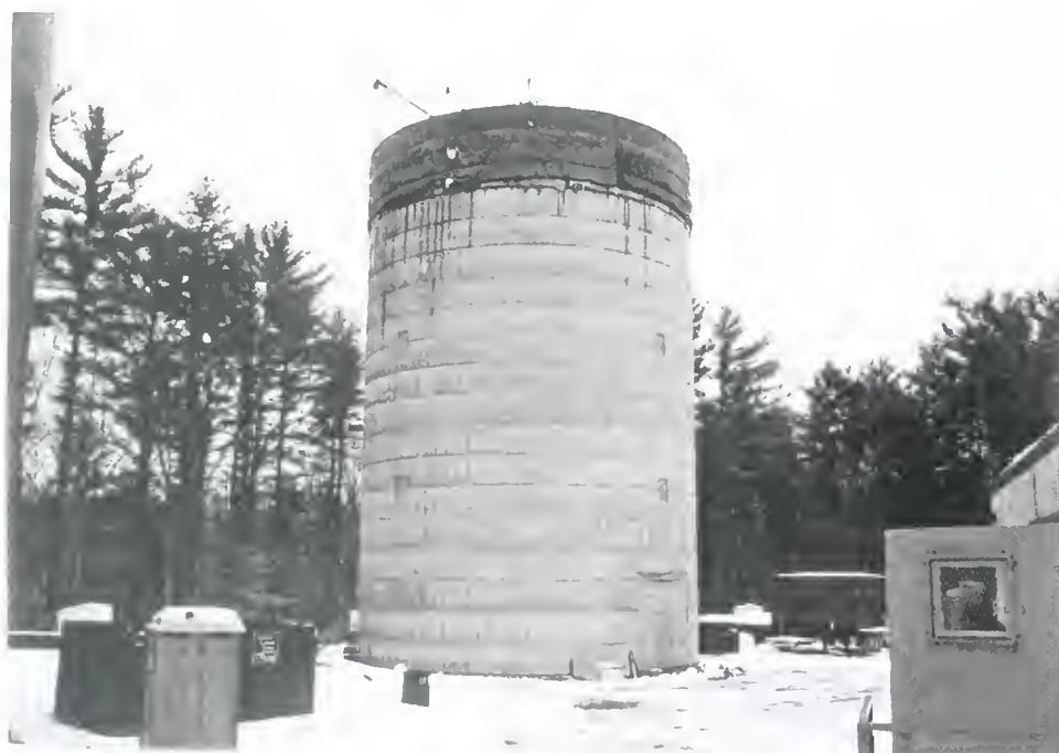
New Epping Road water tank – under construction Dec 2007
